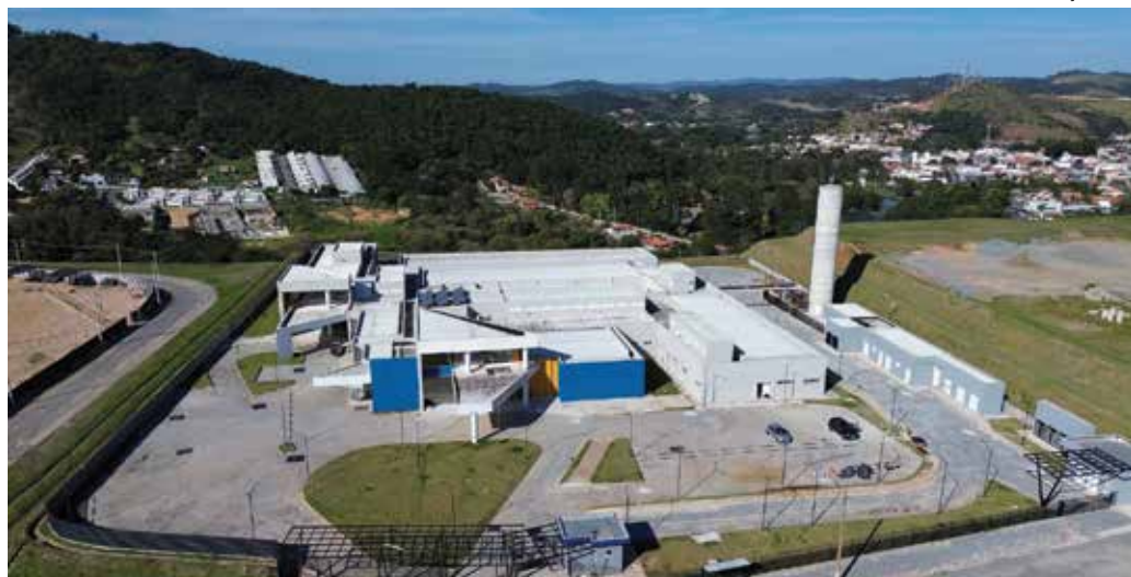
Obra Hospital Municipal
